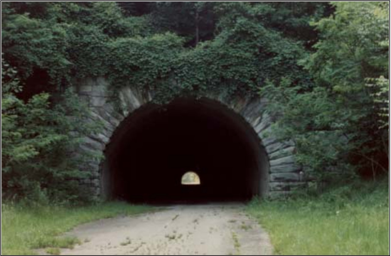
Figure 1.2. Lake View Drive tunnel through Forney Ridge.
