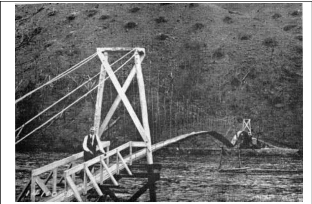
Figure 4.29. The swinging bridge at Bushnell.
