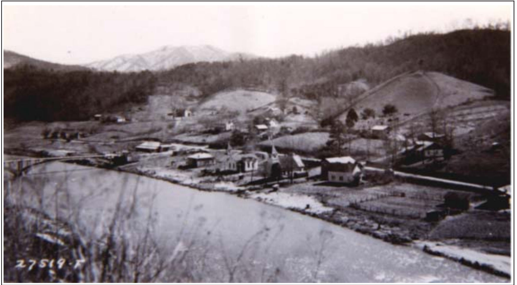
Figure 4.41. Judson (view to northeast).
