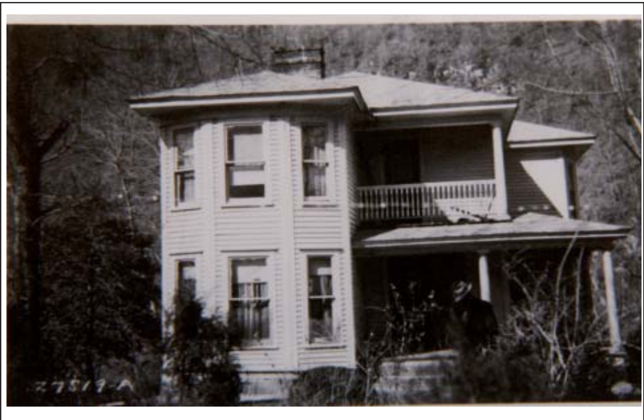
Figure 4.51. Frame house in Fontana acquisition area.
