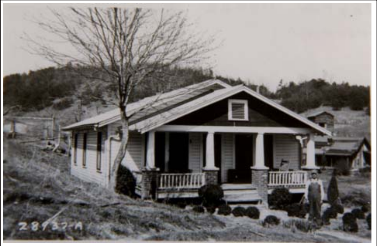
Figure 4.50. Frame house in Fontana acquisition area.
