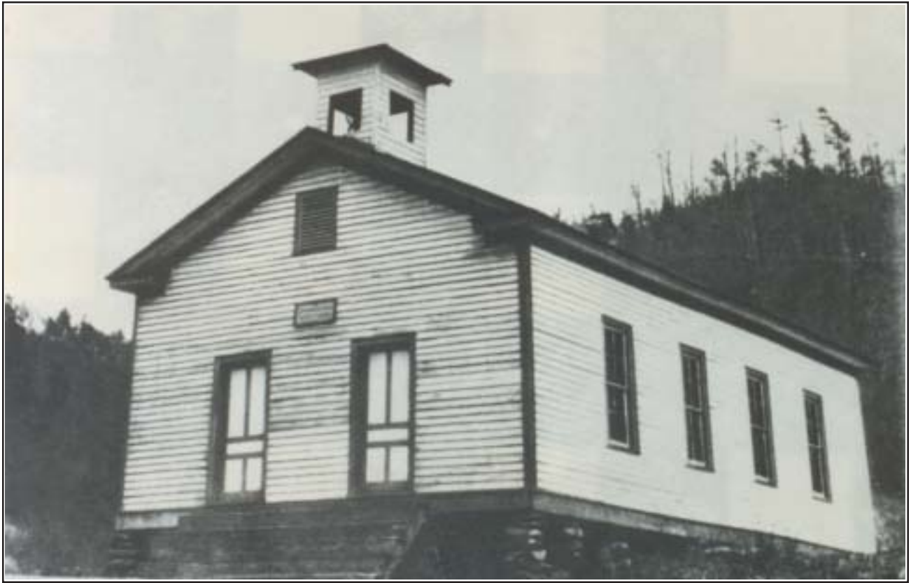
Figure 4.54. Chambers Creek Church.
