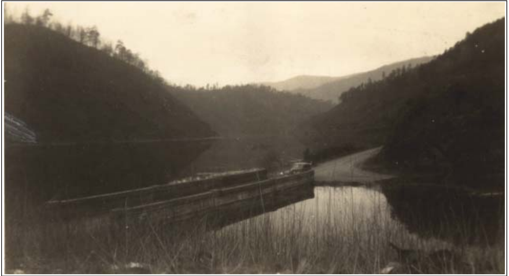
Figure 4.56. Water rising at Forney Creek Bridge.
