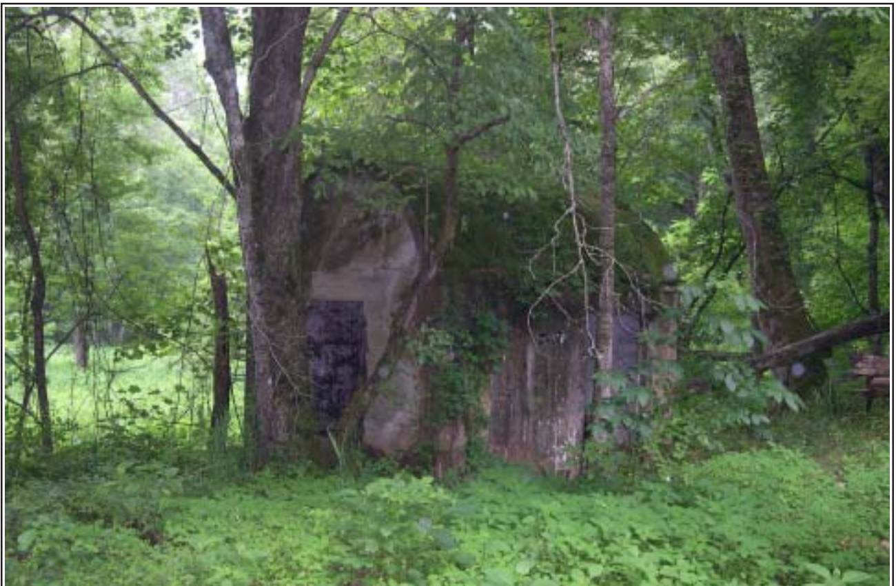
Figure 5.14. Pump or valve house at Proctor.
