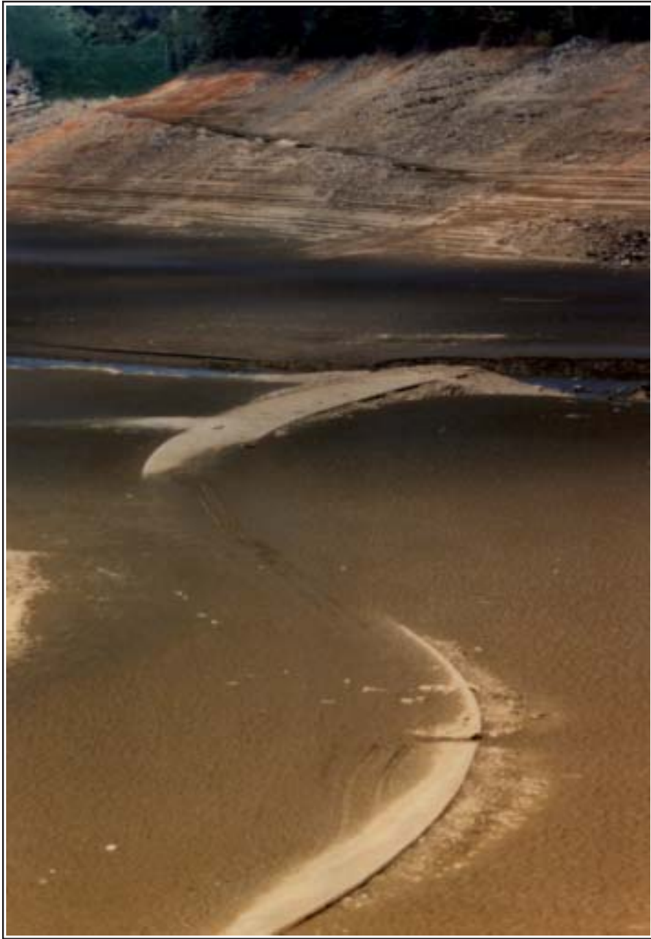
Figure 5.17. Former NC 10 under water at Almond.
