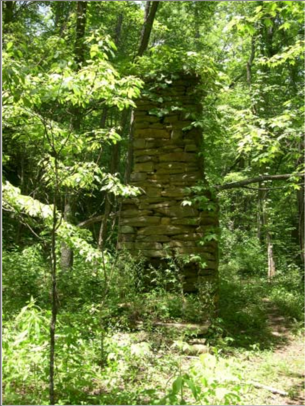
Figure 5.2. Standing chimney at Chambers Creek campsite.
