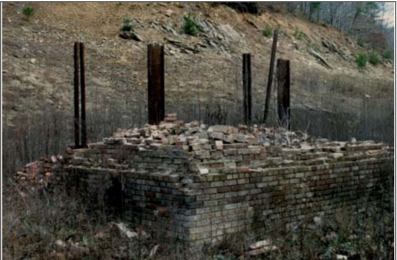
Figure 5.4. Power house foundation at Fontana Mine.
